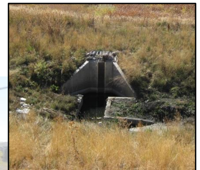
Outlet Structure Example
