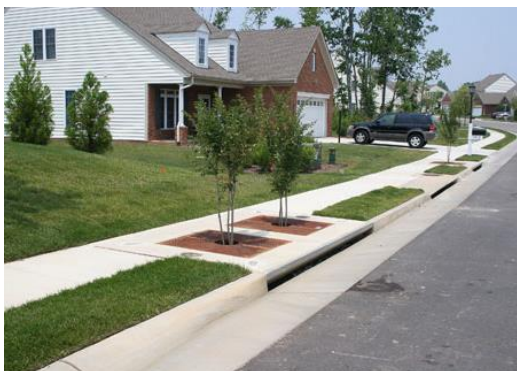
Figure 5. Landscape Filtration Systems Source: Filterra® System
