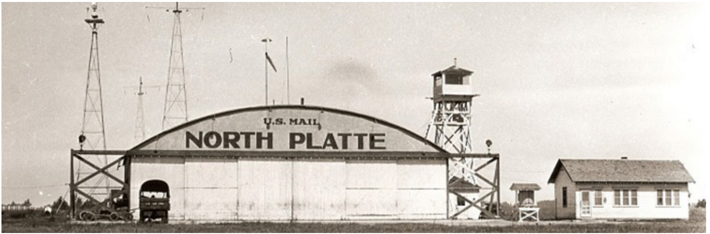
North Platte airport was on the Trans-continental flyway for the delivery of U.S. Air Mail. This circa 1924 photograph shows the airmail beacon on the left on the hangar which played an important role in safety and navigation. To increase the speed of the night delivery of air mail, the post office eventually built a series of lighted beacons ten to fifteen miles apart between Cheyenne and Chicago. (National Postal Museum photograph)
