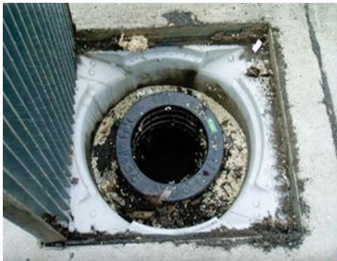
Figure 3. Catch Basin Inserts Source: Triton® Catch Basin Inserts
