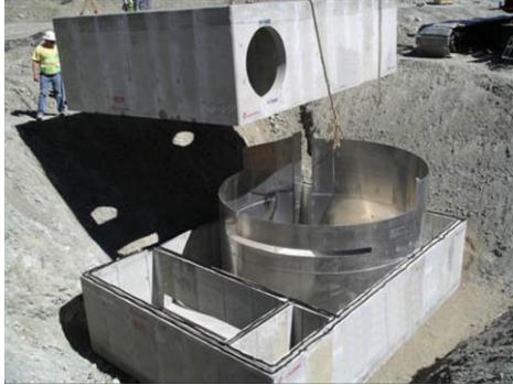
Figure 1. Hydrodynamic Separator Source: Vortechs® System
