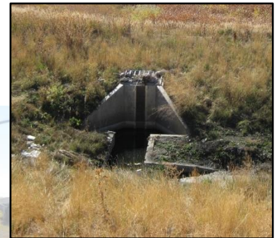
Outlet Structure Example
