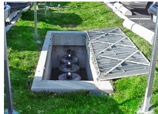
Figure 4. Media Filtration Systems Source: StormFilter® System
