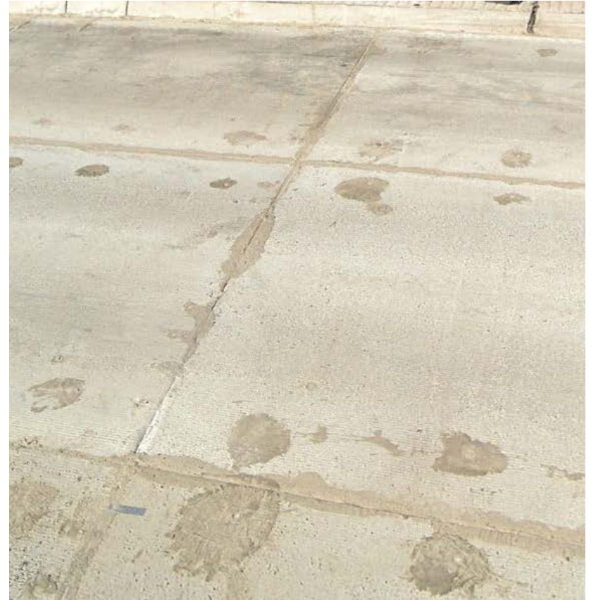
Final concrete repair complete
